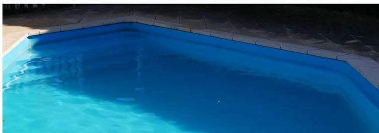
The image above right is of a liner that is only around three years old, but has permanent stains at the water line. There are two reasons for this - poor or irregular maintenance, and excessive use of sun-screen by swimmers - especially P20 cream. Whilst the liner isn't harmed by this, it's unsightly.
